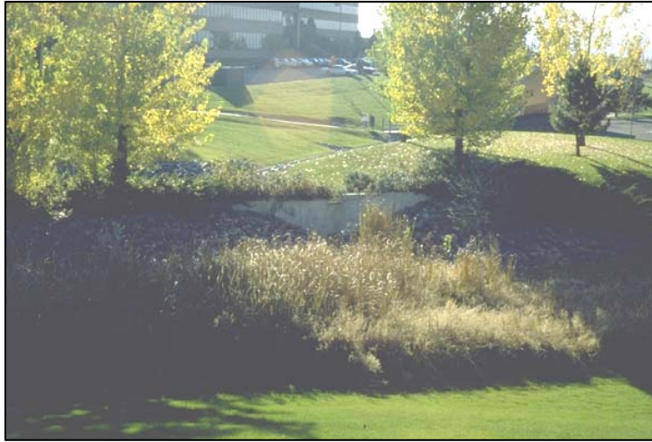
Photograph SO-4—This on-site dry detention facility (note short concrete dam) promotes pollutant removal in smaller runoff events.
