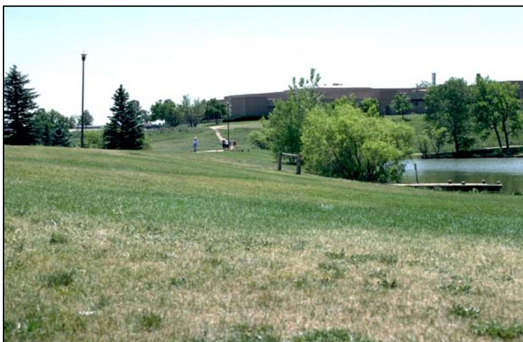
Photograph SO-7—This retention pond has an embankment with upstream and downstream gentle sideslopes, which promotes dam safety and multipurpose use.
