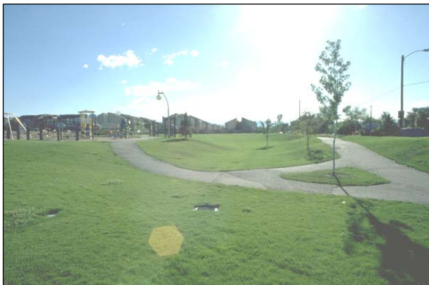
Photograph SO-3—On-site storage facility serving town home development (in background) coupled with park.
